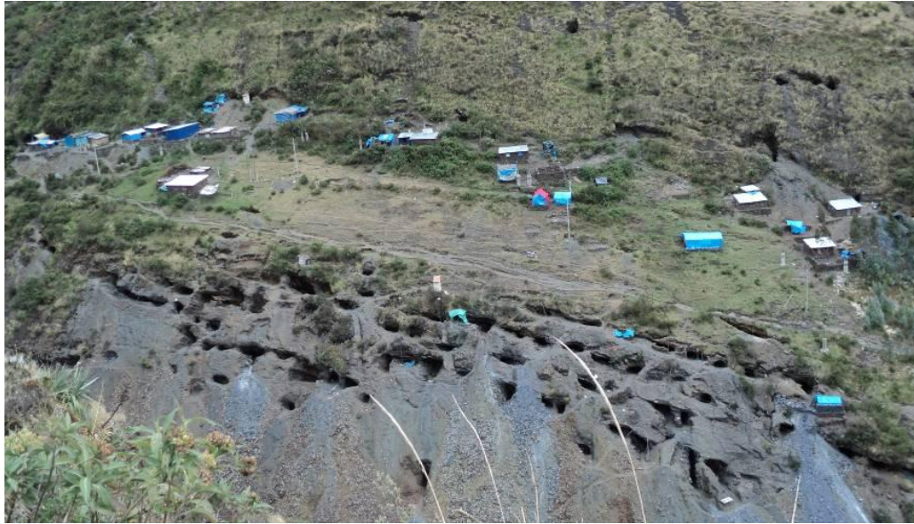
Figure 6-1: Artisanal Mine Workings at Minapampa - October, 2010
