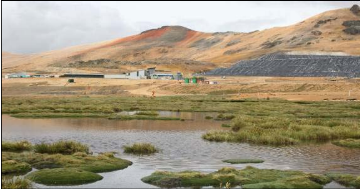
Figure 5 Plant and heap leach, January 2010, showing wetlands in the foreground
